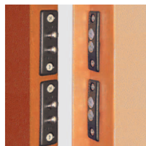
Double electrical contacts between leaf and doorframe
